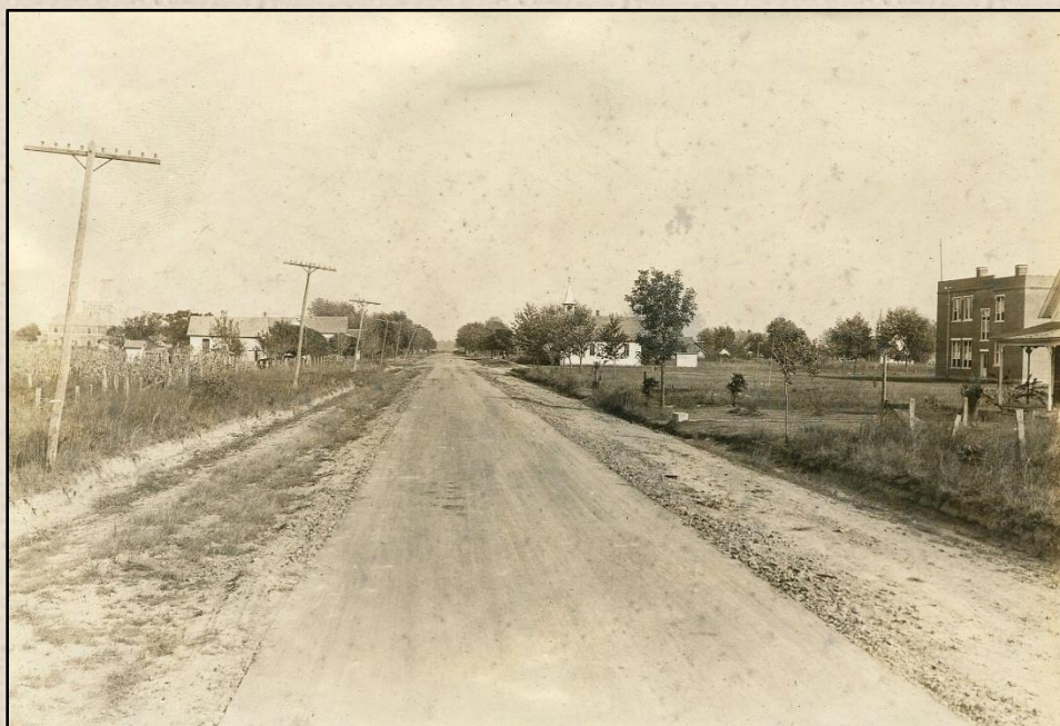
Early road paving in Almyra, Arkansas. Courtesy of the Museum of the Arkansas Grand Prairie.
